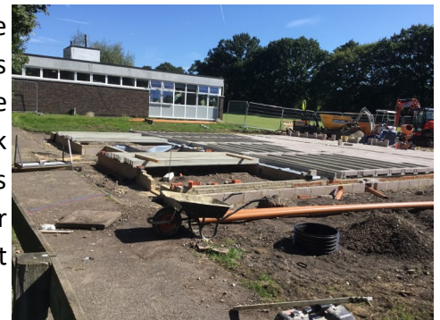
The progress of our new building
